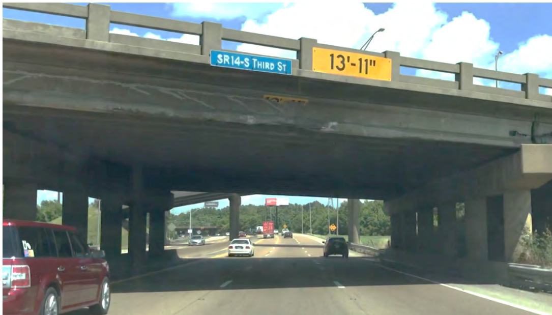
I-55 approach, looking eastbound, clearance 13'11", damage
